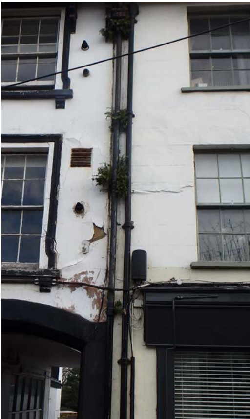
Blocked and overflowing downpipe
