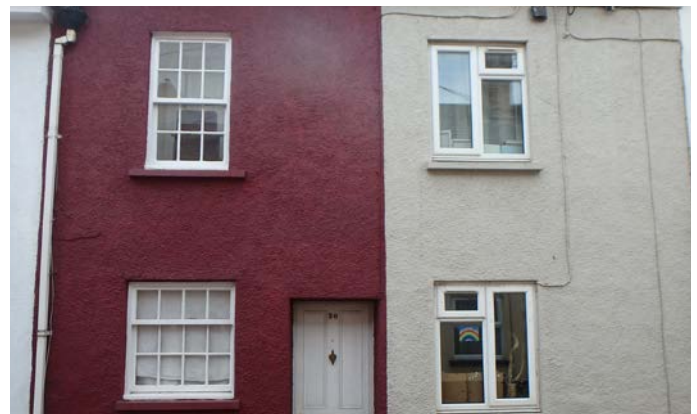
Original and replacement windows side by side
