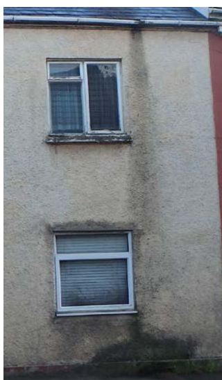
Long term damage from poorly maintained rain water goods
